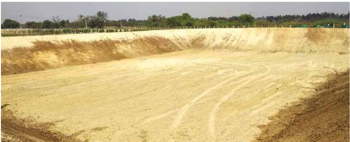
Under-construction rainwater harvesting pit
