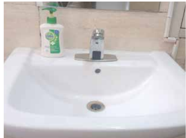
Sensors installed in the taps of washroom
