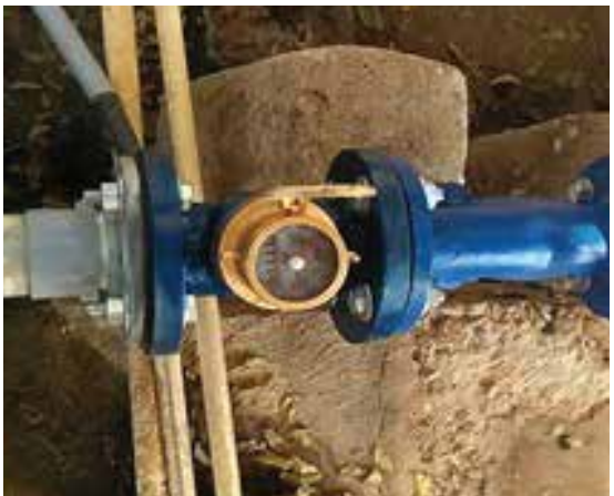
Installation of water meter for monitoring
